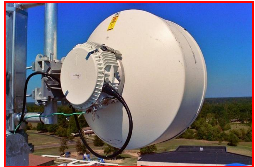
Outdoor Unit Directly Mounted to Antenna
